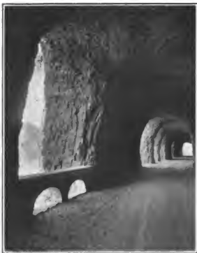
TUNNEL AT MITCHEL'S POINT
